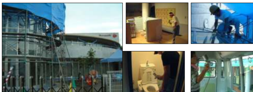
Exterior concrete, and entrance glass windows. Location : Numazu city, Shizuoka prefecture.
