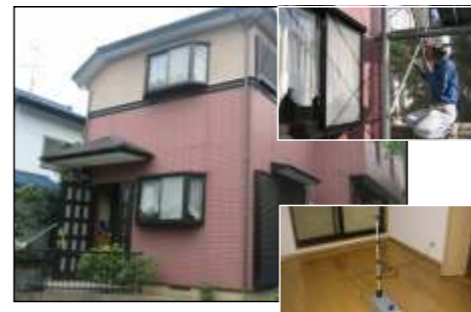
Exterior and interior. Location : Kawasaki city, Kanagawa prefecture.
