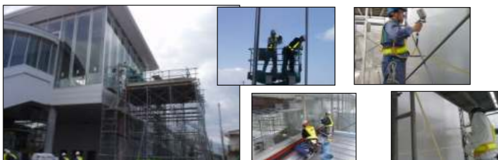
Exterior wall panels, Glass windows. Location : Nagano prefecture.
