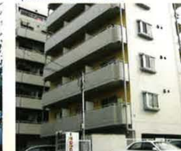
Appearance can be maintained, which improves the occupancy rate
