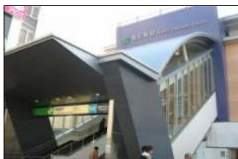
Exterior wall Location : Chiba prefecture.
