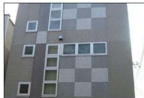
Exterior wall tiles. Location : Kanagawa prefecture.
